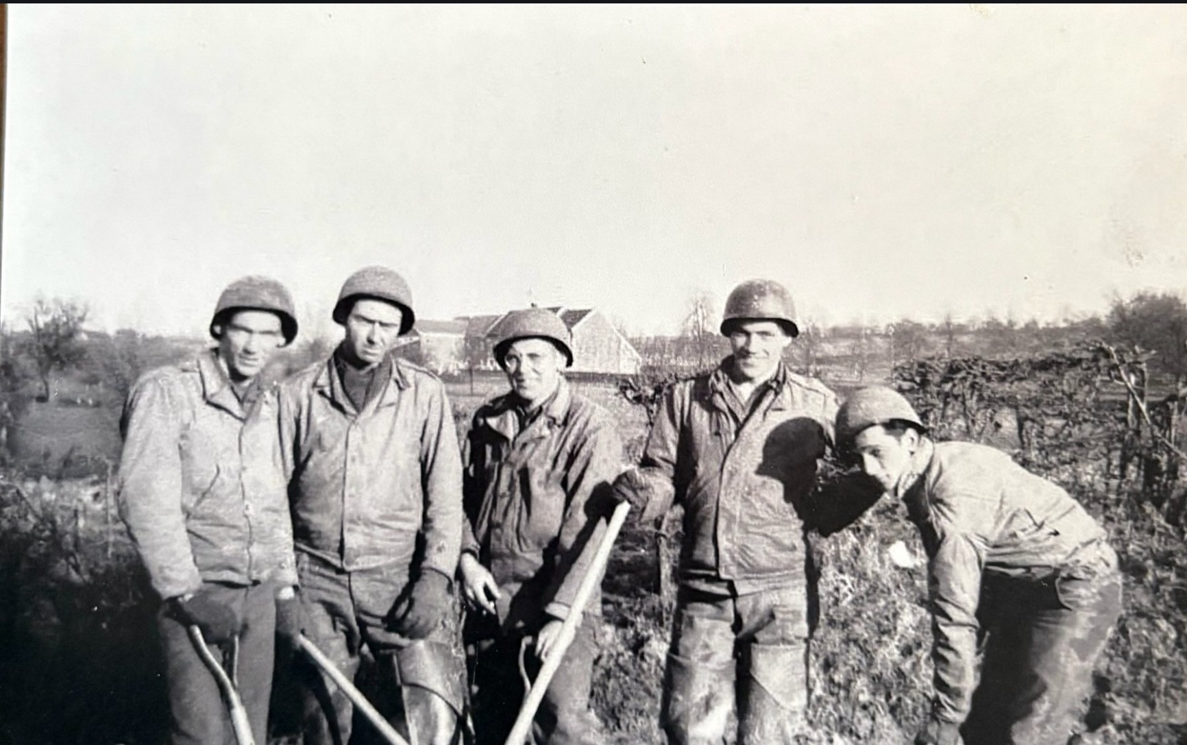
George (far left) with his engineer squad and their shovels, a European farmhouse behind — exactly the road-and-bridge work the letters describe. In a letter from this stretch George mentions a photographer snapping them building a bridge. (Autumn 1944 · France or Belgium (likely))
